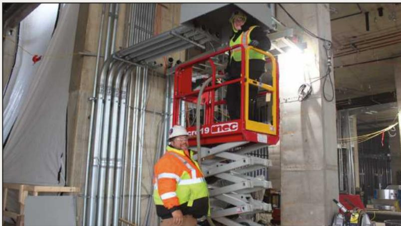
PULLING STRING as a method to measure conduit on the first level of the Gun Lake Casino hotel under construction in Wayland are Dan Damick and Tony Falvo (on the left) of IBEW Local 131. They're employed by Moore Electric.
