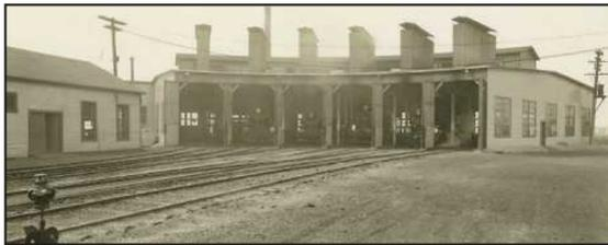
THIS ROUNDHOUSE IN Flat Rock served Henry Ford's Detroit, Toledo and Ironton Railroad. It is shown in 1924. The DT&I operated a 378-mile mainline between Detroit and Ironton, Ohio. While the structure has been demolished, the turntable that was inside is intact, reports SteamLocomotives.com.
